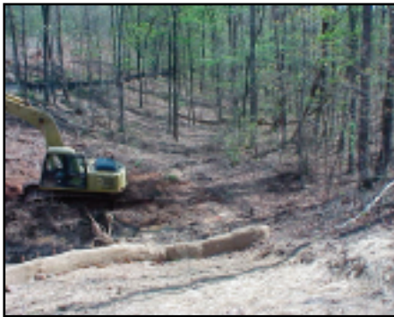
During excavation the site was stabilized with polymer enhanced soft armoring.
