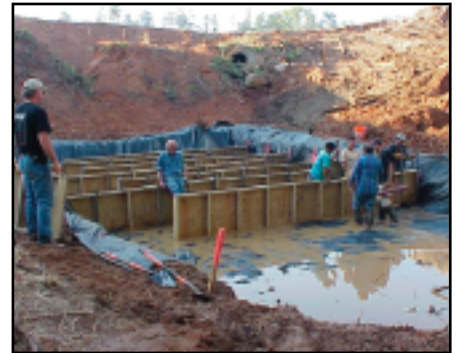
By constructing a floc log mixing chamber, a baffle grid, the water can be channeled through the system creating the mixing required to allow the system to react and the particulate to flocculate out.
