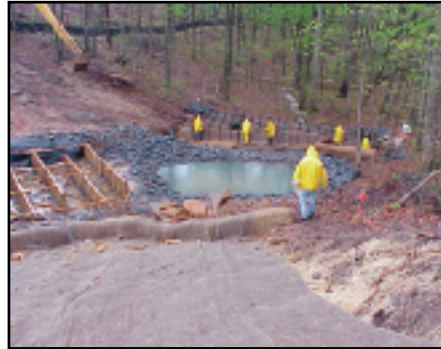
The baffle grid is for use in conjunction with a stormwater treatment system to flocculate the suspended particles, making larger particulate that can easily be removed from suspension.
