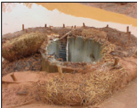
An inlet sediment trap is used to prevent silt from entering the pipe system at an inlet.
