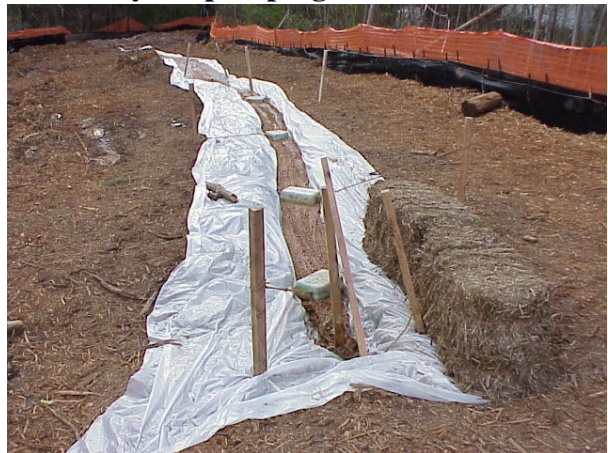
6) Ready for pumping
