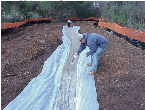
5) Apply Silt Stop (downstream end)
