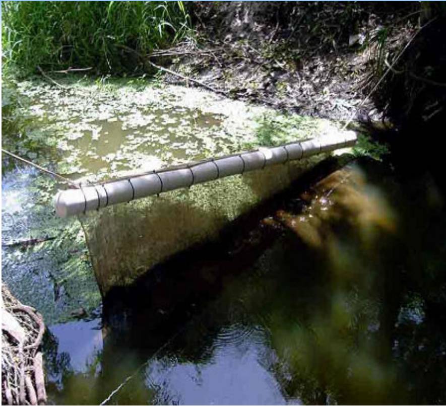
Above: Particle curtain strategically placed to catch the particles that did not settle out by gravity.
