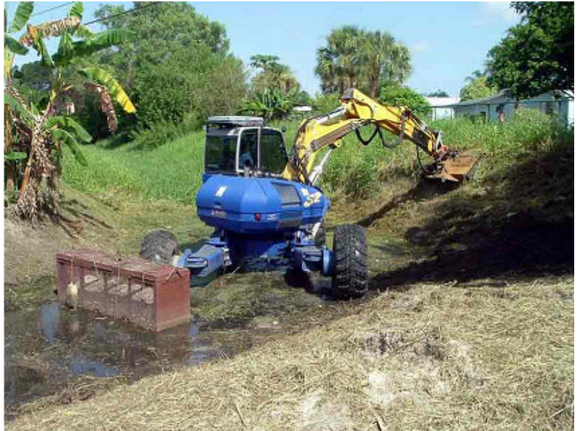
Design: A movable metal box was designed for ease of mobility and mixing of the Floc Logs. Note the Floc Logs placed within the metal box.
