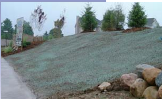
After 1" rainfall in October 2001
