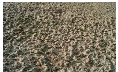
Mulch condition on slope after 1" rainfall
