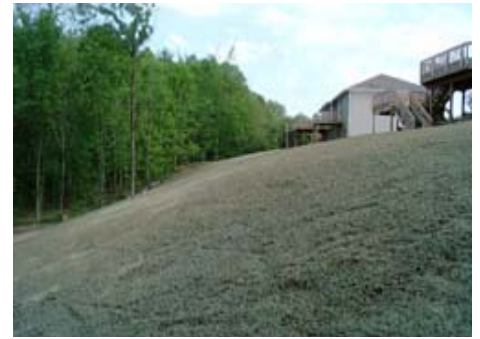
Mulch condition on slope after 1” rainfall
