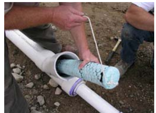
Insertion of Floc Log into wye element
