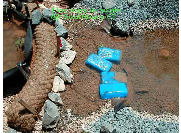
Floc Log ditch placement, used in conjunction with BMP's
