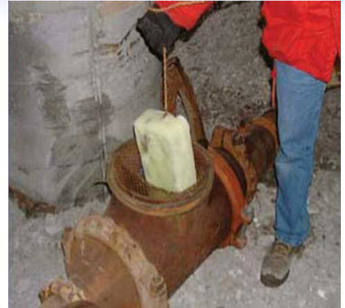
Floc Log placement in a pipe system
