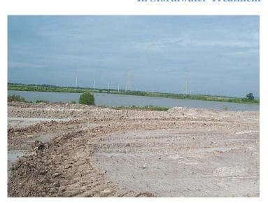
The rains had carried excess sediment into the retention ponds, causing turbidity problems. The excess water needed to be removed quickly, which did not allow time for the sediment to settle out of the stormwater. In fact the dewatering operations would stir up the sediment, causing elevated turbidity in the ponds and in the water to be discharged.
