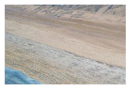
Jute matting was installed at the end of the treatment ditch system and applied with the APS 705 Silt Stop powder. The jute matting provided a surface for the flocculated particles to adhere to and the 705 powder helped capture the fines still in suspension.
