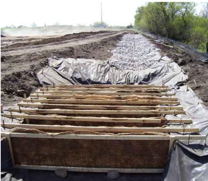
The turbid water mixed with the Floc Logs as it traveled down the ditch line, allowing the polymer to dissolve and react with the suspended sediment, binding it together and causing it to drop out of suspension.
