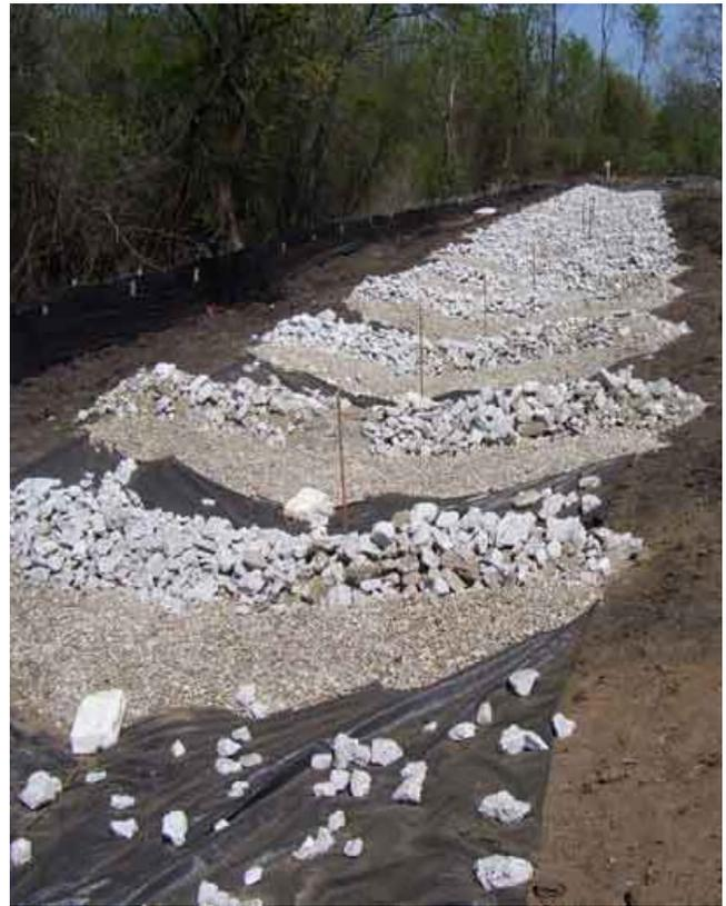
A continuous flow-through treatment ditch was designed for use with site-specific polymers to address the turbidity problems on the site. The stormwater was kept in the retention pond while the treatment ditch and baffle system was constructed and then pumped into the treatment system. The ditch was lined with a geotextile fabric then rip-rap and filter stone were installed into the swale.
