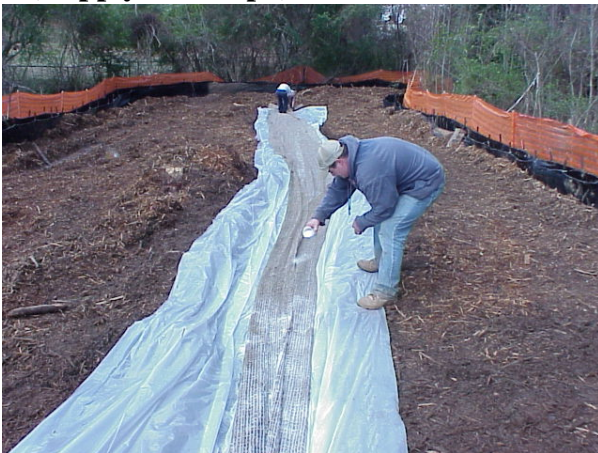
5) Apply Silt Stop (downstream end)
