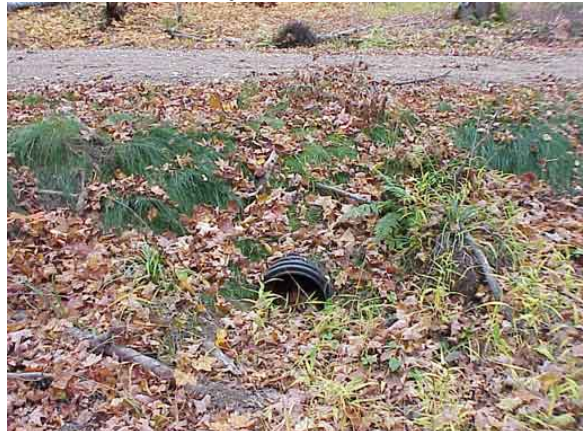
6) Stabilized 1 year later
