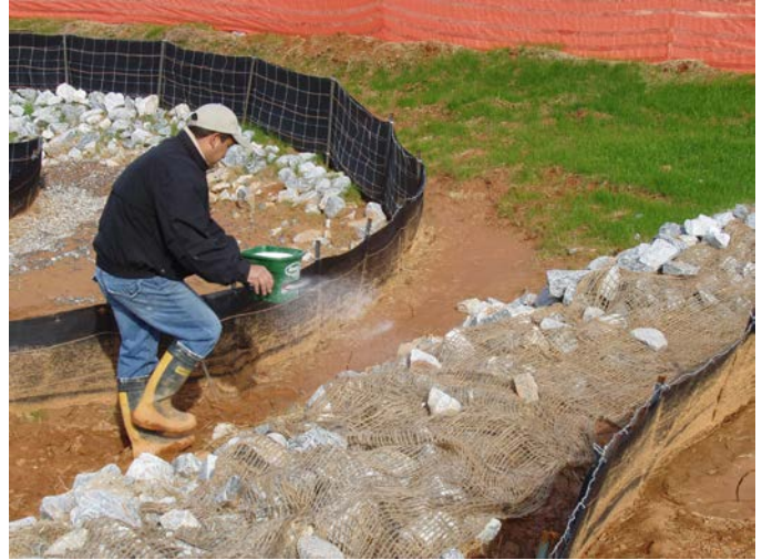
Apply Silt Stop powder over rock check
