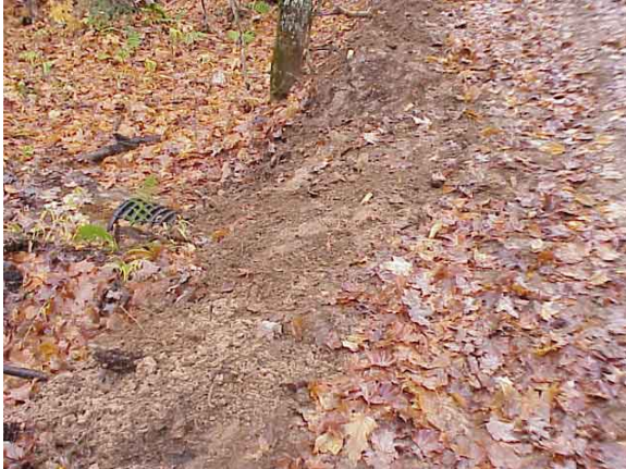
1) Fill rills and gullies
