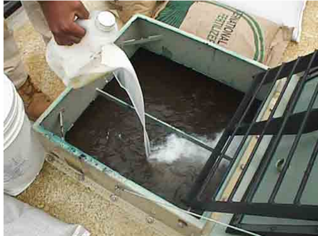
4) Add Silt Stop as final additive to mix
