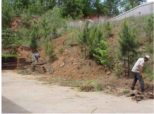
2) Fill rills and gullies
