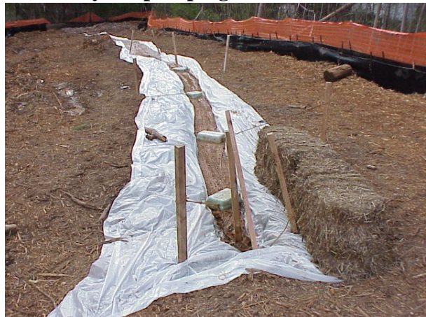
6) Ready for pumping
