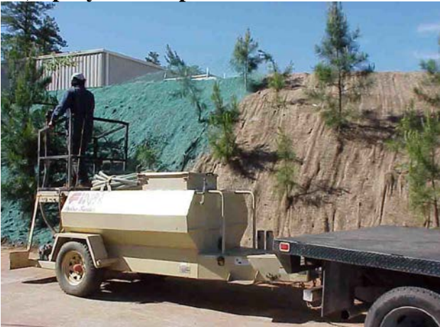
5) Spray onto slope
