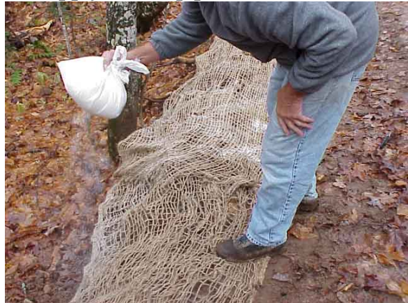
4) Apply Silt Stop powder
