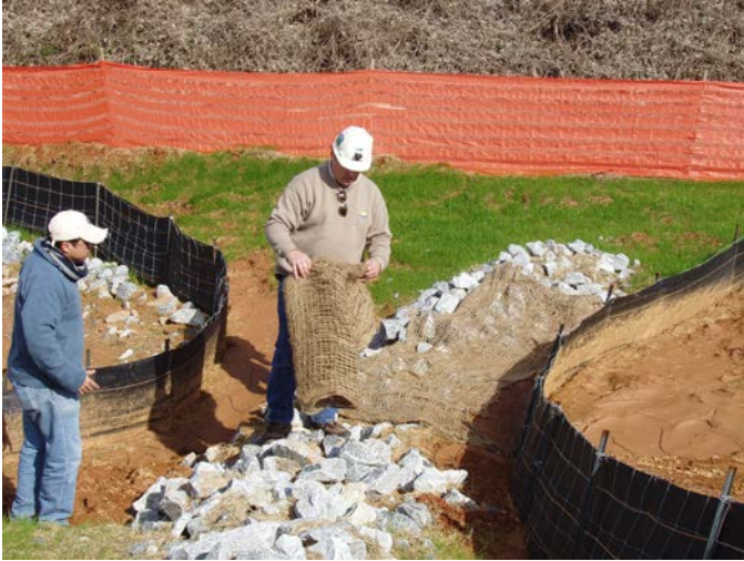
Cover rock check with jute matting
