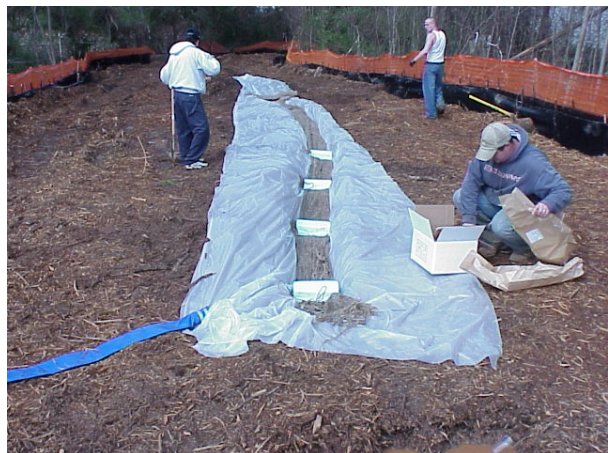
4) Place Floc Logs (upstream end)
