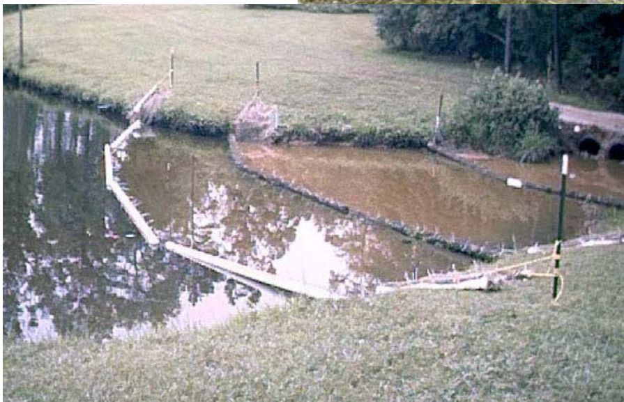
(Left) A series of particle curtains collect suspended flocculated material resulting in progressively clearer water.
