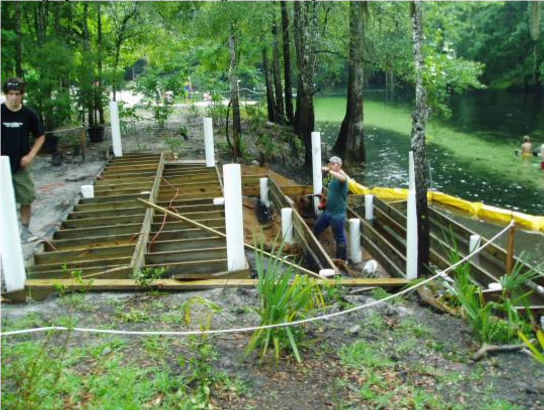
Photograph 10. June 21, Decking and cantilever steps
