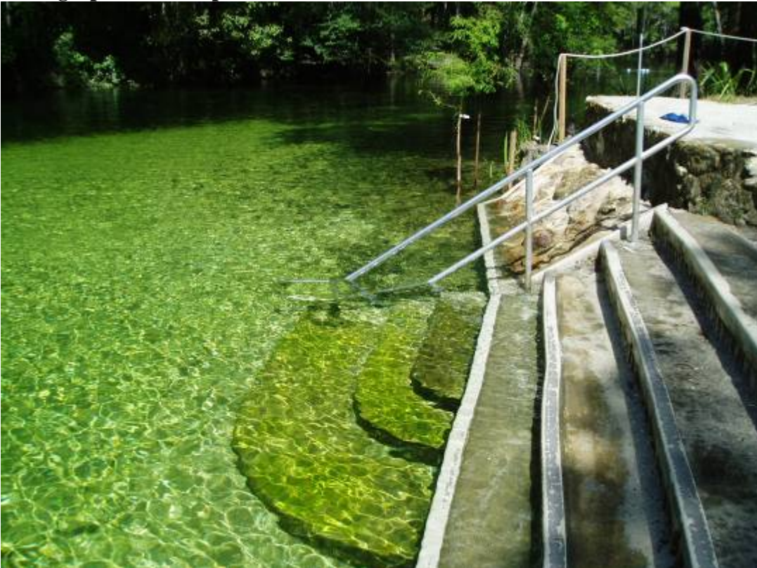
Photograph 17. Completed concrete stairs
