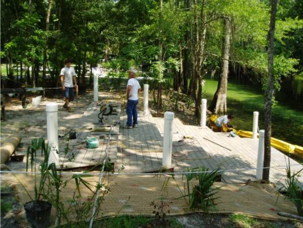
Photograph 11. June 23, Decking finished, handrails begun, jute fiber mat installed
