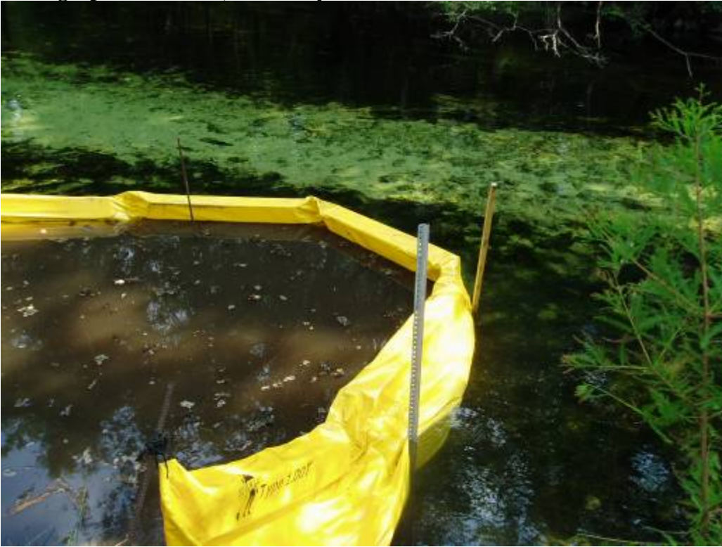
Photograph 7. June 15, Turbidity curtain
