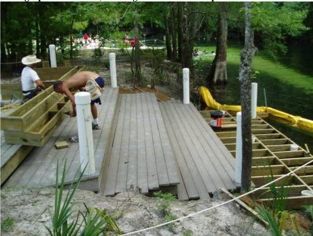
Photograph 10. June 21, Decking and cantilever steps
