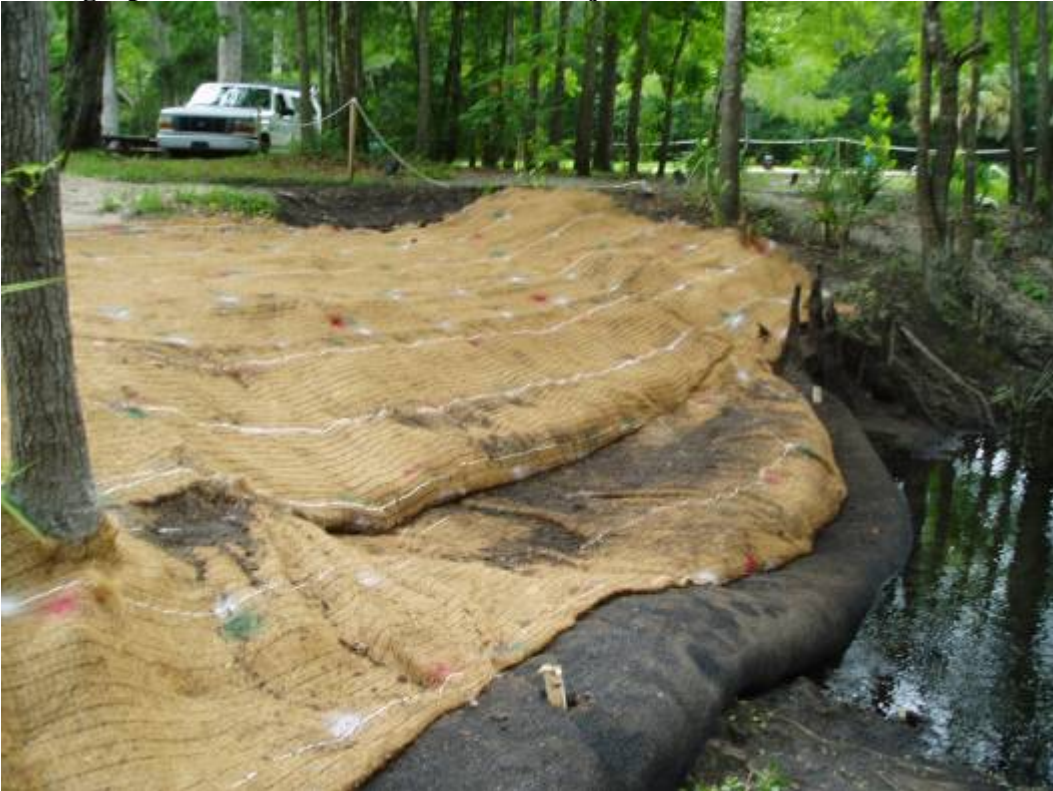
Photograph 3. June 10, Filtrexx socks and jute fiber mat
