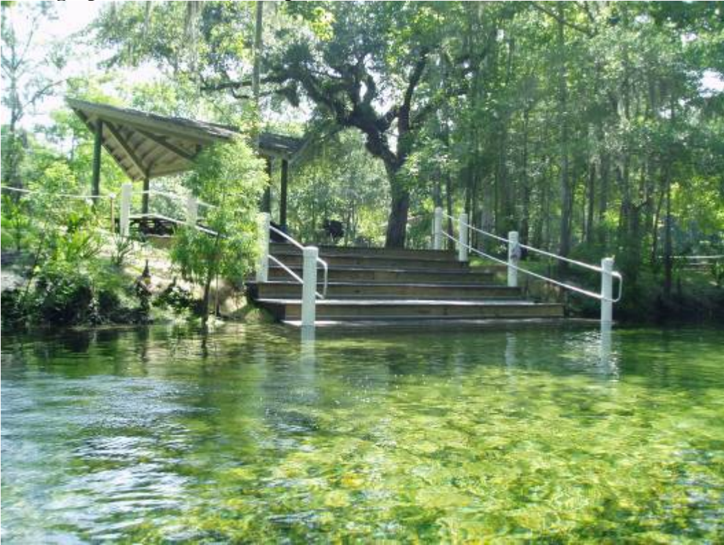
Photograph 16. June 30, Completed Staircase
