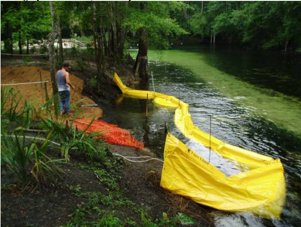
Photograph 4. June 13, Turbidity curtain
