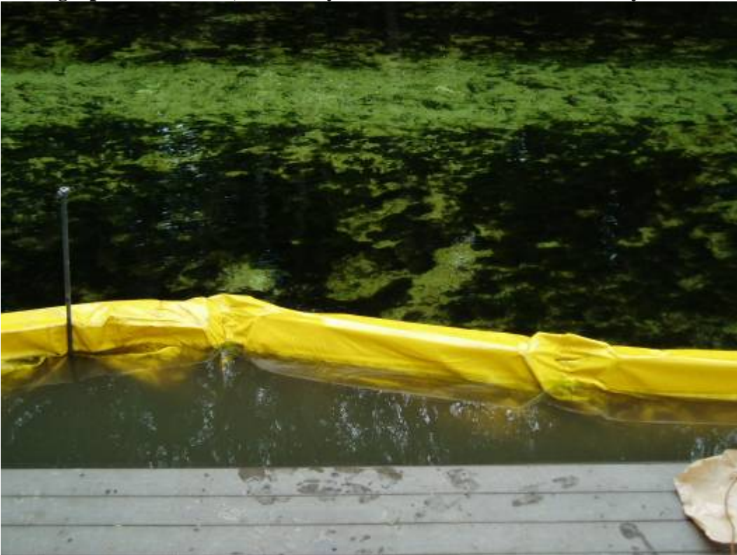
Photograph 12. June 28, Turbidity inside and outside the turbidity curtain
