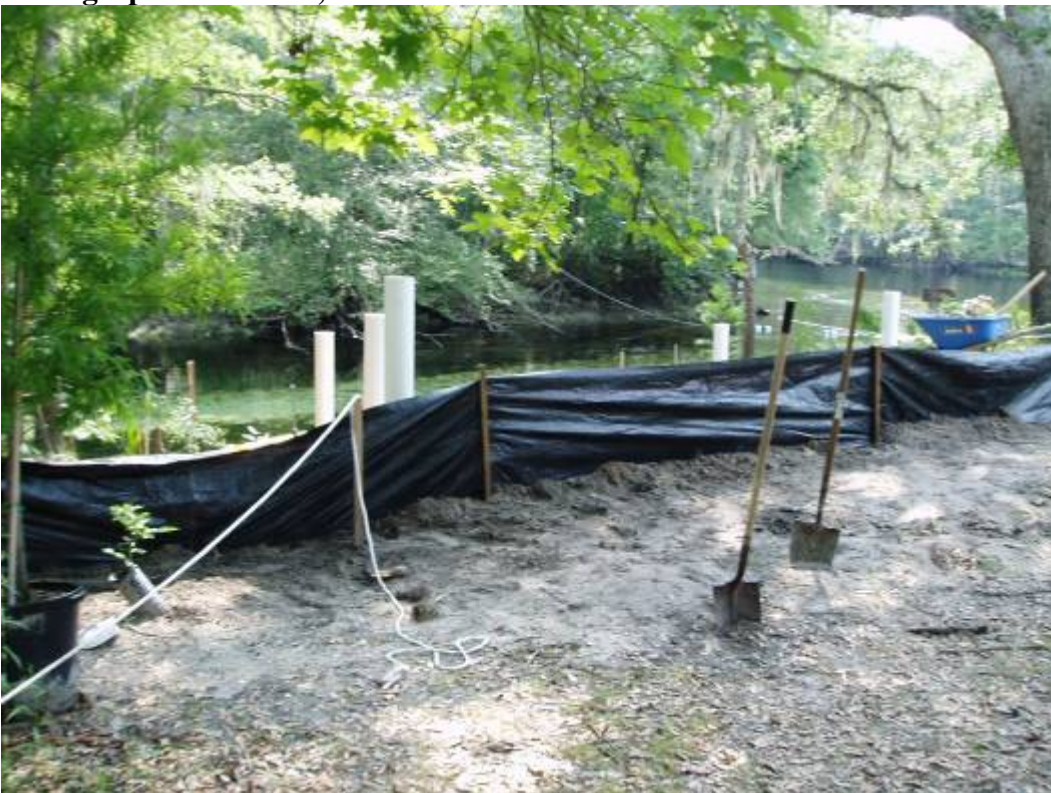
Photograph 8. June 15, Silt fence
