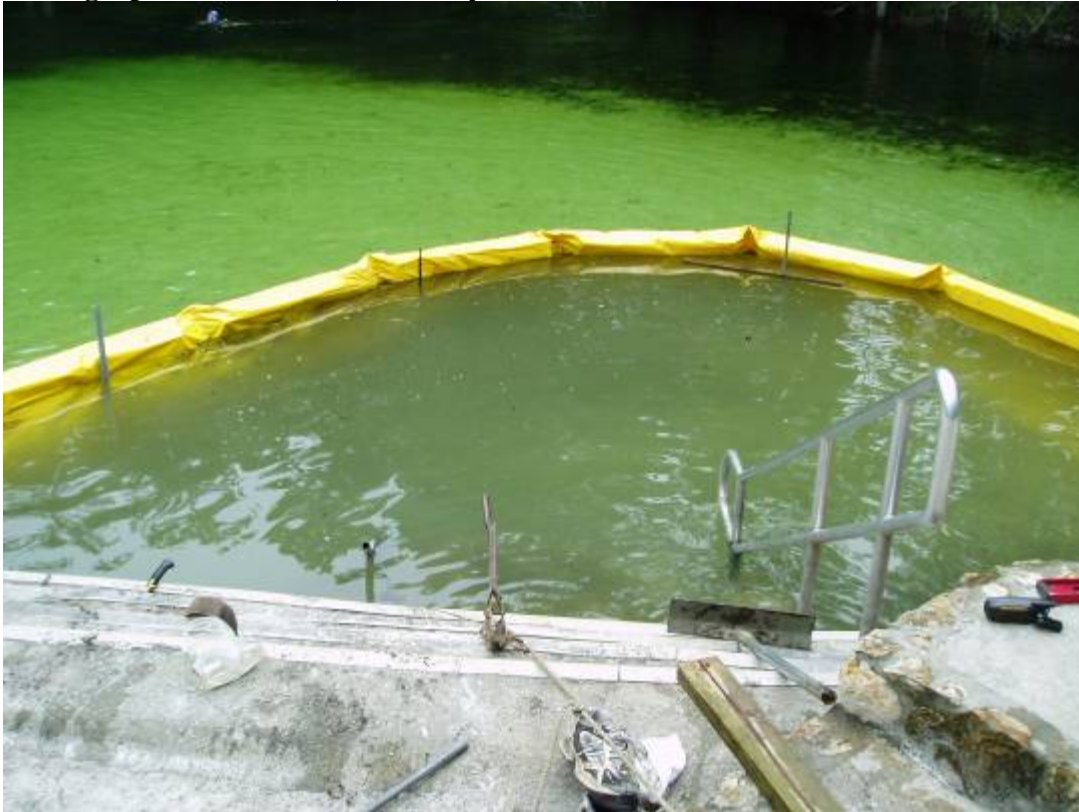
Photograph 13. June 28, Turbidity curtain for staircase installation
