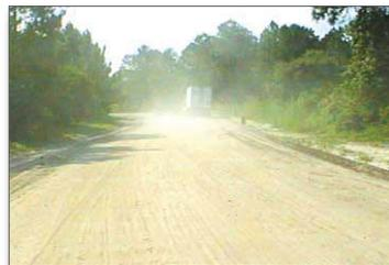
Figure 12. Road dust before applying polymer flocculant
