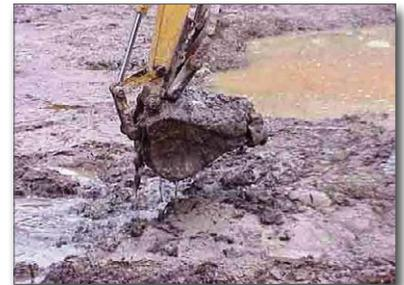
Figure 36. Removing stiffened sediment from a sediment basin
