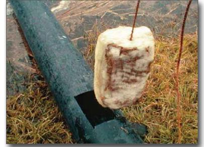
Figure 19. Polymer blocks inserted into pipes
