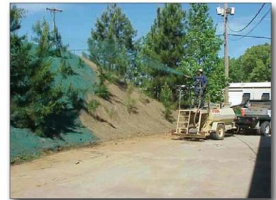
**Figure 5.** *Hydroseeding the slope*
