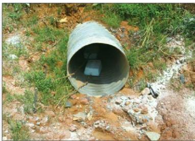
**Figure 39.** Polymer block in a construction site culvert
