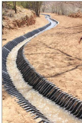
Figure 18. In-ground treatment ditch
