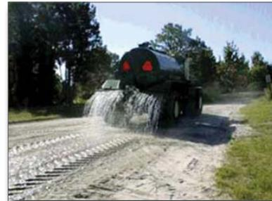
Figure 11. Water truck applying dissolved polymer flocculant
