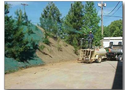
**Figure 5.** *Hydroseeding the slope*
