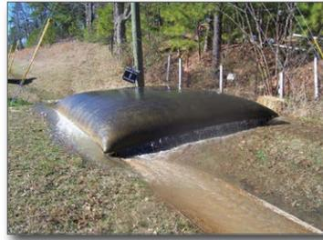
Figure 34. Sediment bag and its treatment ditch
