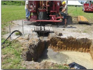
Figure 7. Drilling rig and settling pit
