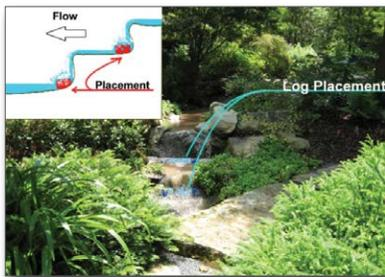
Figure 32. Polymer flocculant logs placed in the waterfall
