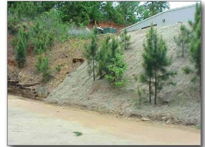
**Figure 4.** *Slope covered with floc collection matting*
