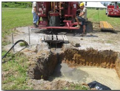
Figure 7. Drilling rig and settling pit
