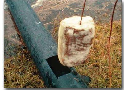
Figure 19. Polymer blocks inserted into pipes
